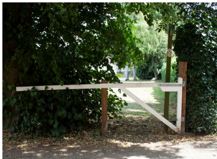
Existing boom swing gate at entrance to pavilion car park
